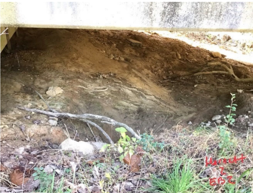
EB2 slope protection: 32' X 40' X 4'
