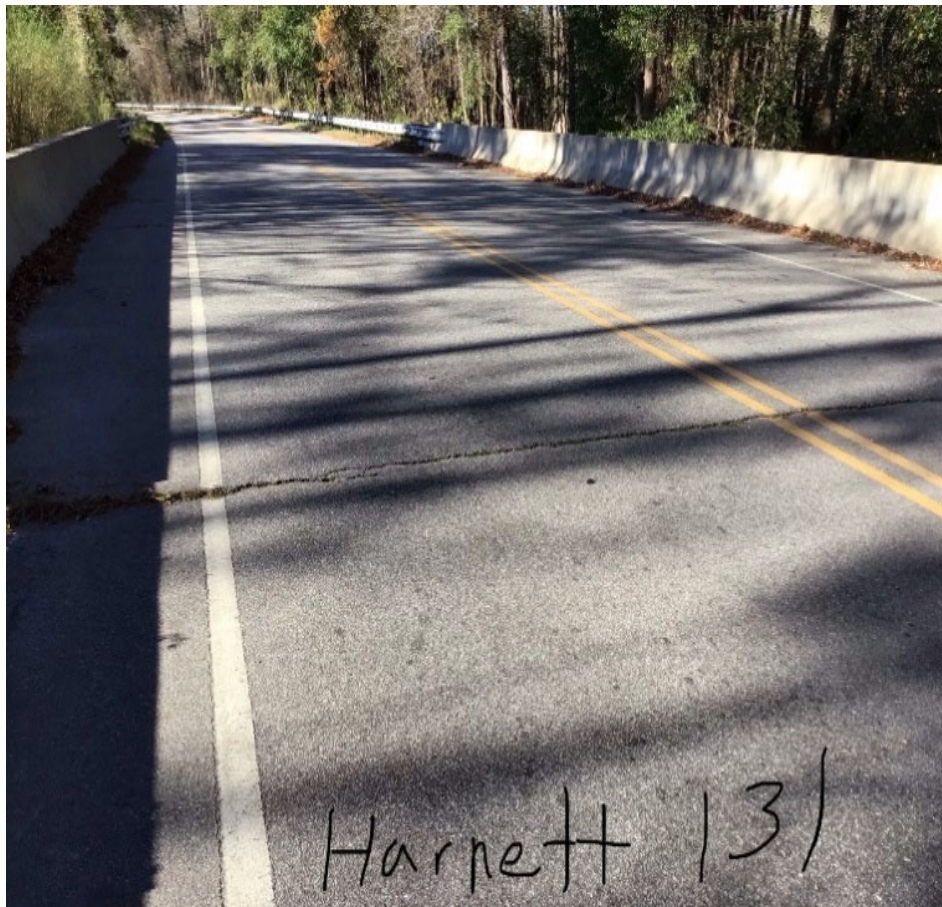
Slab Jacking with Polyurethane foam injection.
